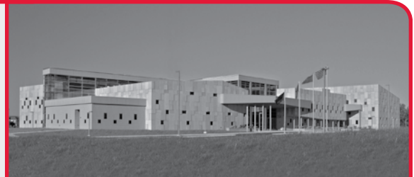
Photography courtesy of SchenkeShultz Architecture
